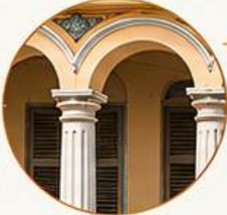
Arches and columns Semicircular arches and classical columns with colonial influence
