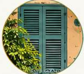
Wooden shutters Louvered doors and windows for natural ventilation
