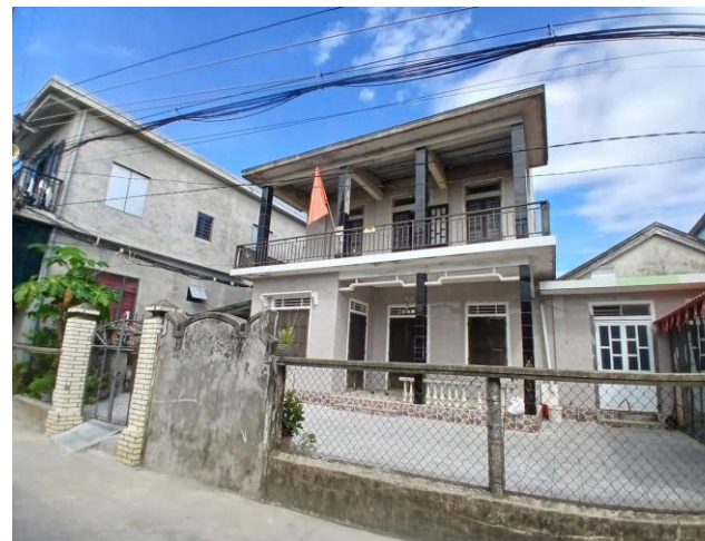
Fig. 12. Raising floor elevation and adding vertical floors for flood resistance (Source: Authors)
