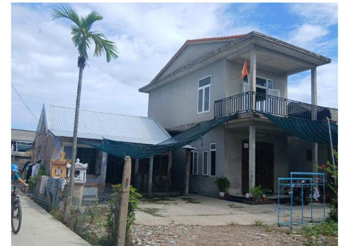
Fig. 12. Raising floor elevation and adding vertical floors for flood resistance (Source: Authors)
