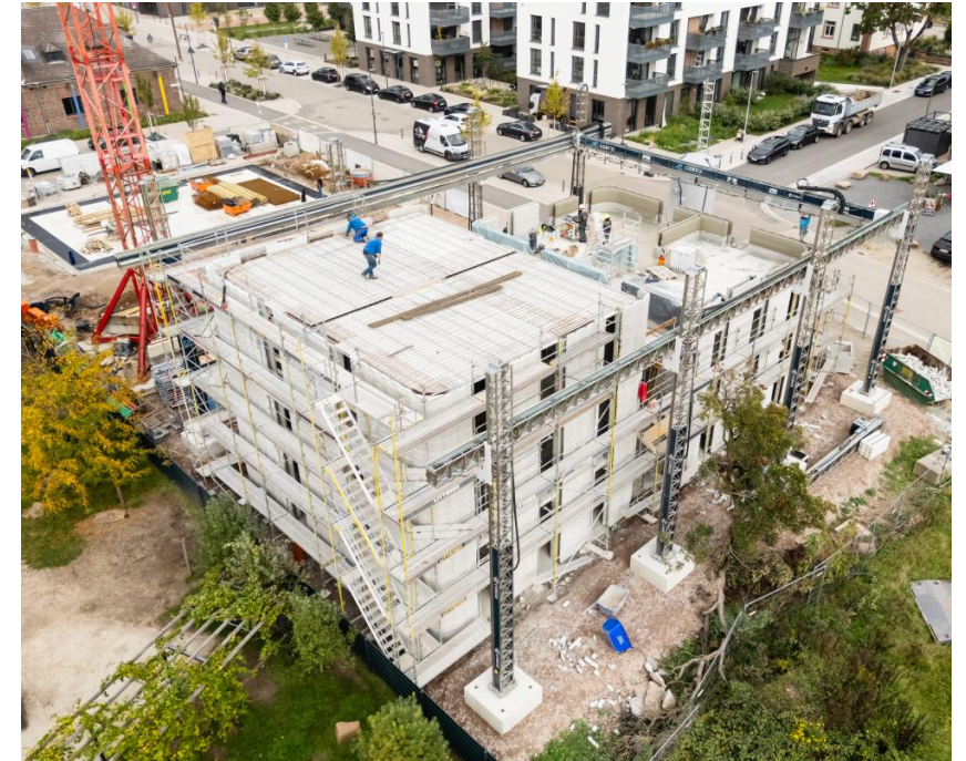
3D-printed residential building in Heidelberg BFT, n.d., https://www.bft-international.com/en/artikel/germanys-first-serially-produced-3d-printed-residential-building-celebrates-its-premiere-in-heidelberg-4309212.html
