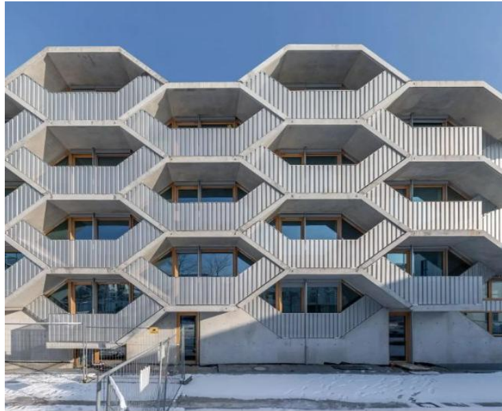
Precast concrete modules for honeycomb house in Germany BUILD OFFSITE, 2024, https://builtoffline.com.au/news/precast-concrete-modules-for-honeycomb-house-offer-alternative-vision-of-architectural-innovation/
