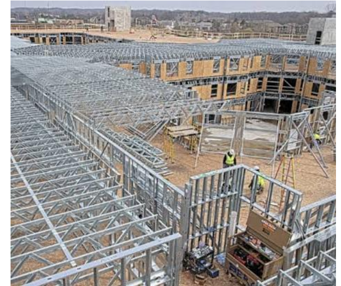
Vista at Brighton, cold-formed steel (CFS) framing. BuildSteel, n.d., https://buildsteel.org/projects/multi-family-residential/intellisteel-converts-wood-framed-project-to-steel/
